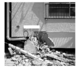
Fig. 2 Failure of beam-column joint
